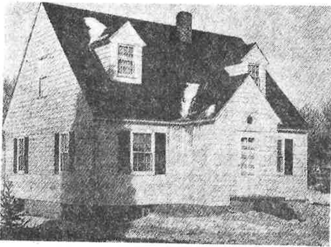
Six-room frame home of C.E. Johnson, Polk county deputy sheriff.
