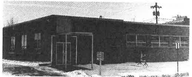
Present Post Office located at 405 Third Street
