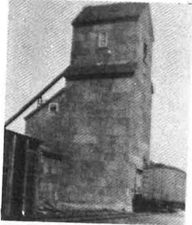
Fire Burns Elevator
