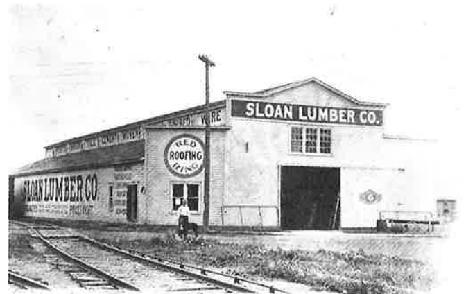
Built in 1912 by J.H. Woods when the yard was re-located on the south side of Third Street west of tracks, 603 Third Street.
