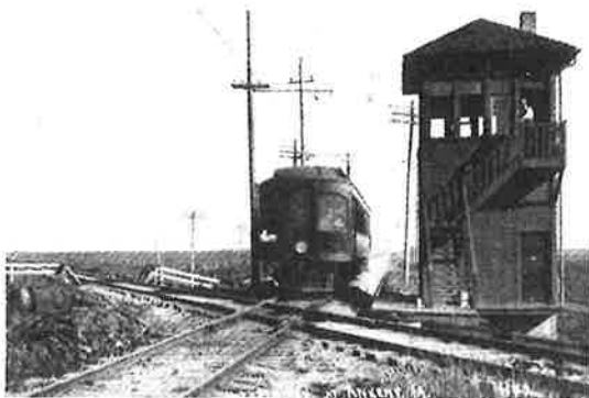
Interlocken station just north of First Street was used when the original track crossed the Northwestern tracks.
