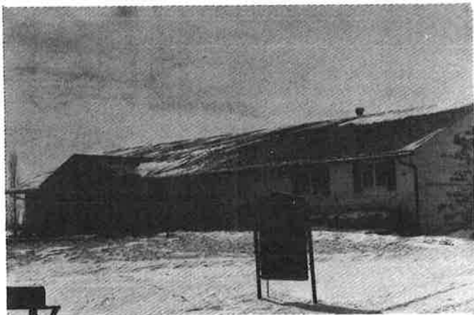
Present church located at 7384 N.W. 16th Street
