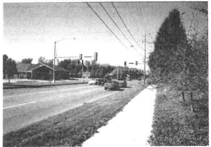
First Street widening was heateaty protested, but eventually won voter's and driver's approval.
