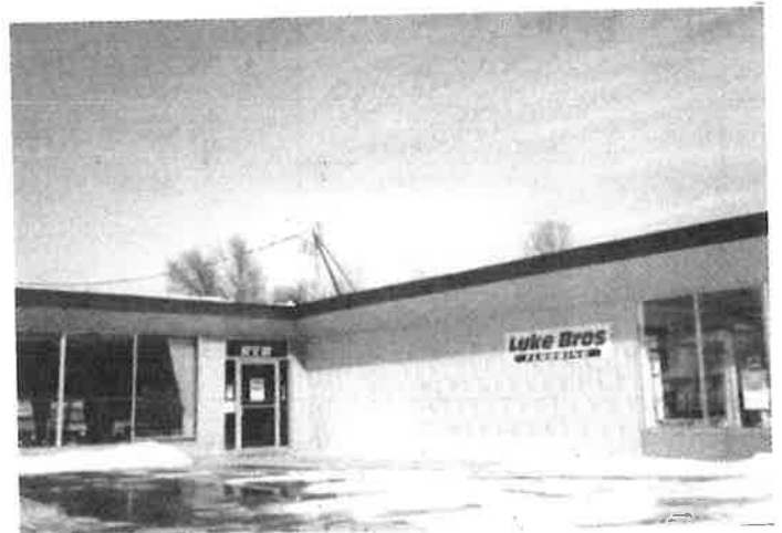
Although their building was once a great hang-out for kids as Toy Villa in the sixties and the tornado of 1974 tried to blow them away, Luke Brothers Carpet has been a generational mainstay of Ankeny. It is one of a handful of businesses that has remained relatively unscathed over the past 30+ years.
