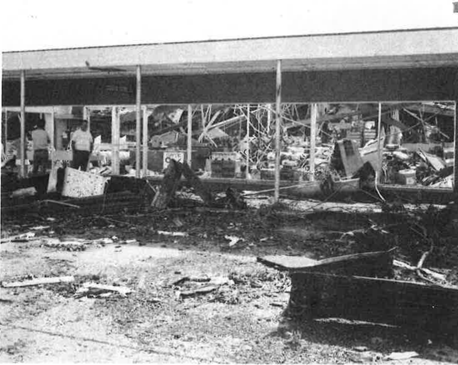
Cory's hardware section was completely demolished, but some appliances were salvaged.
