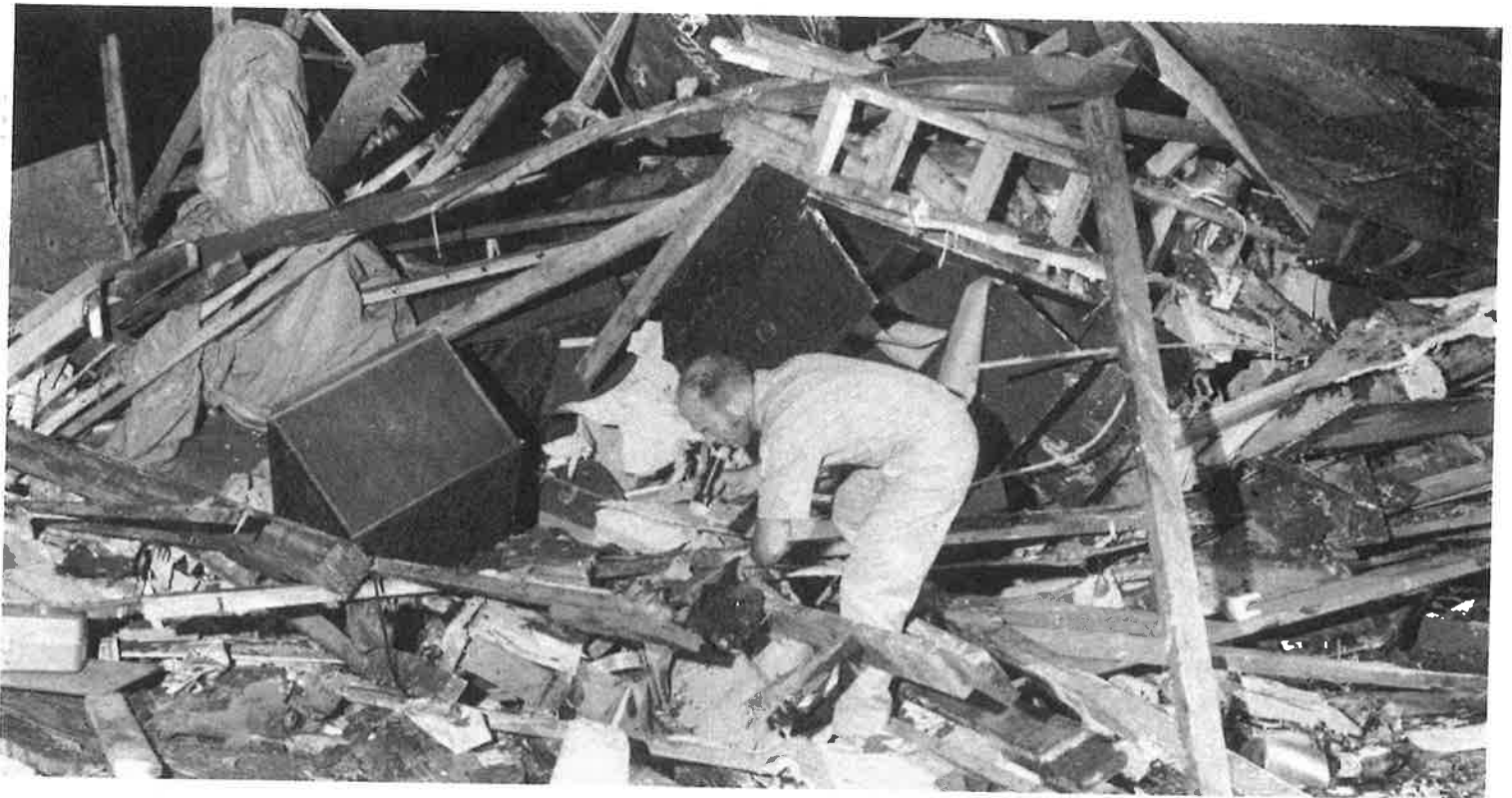
Jerry Card, Ankeny Safety Director pokes through rubble of the home at 1110 Trilien Dr. where Mr. and Mrs. Wallace White were killed and their house was demolished.
